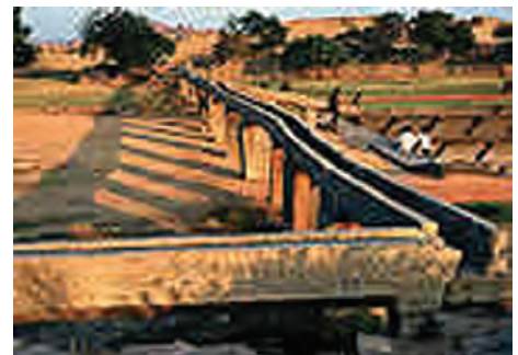
Fig. 7.5 An aqueduct leading into the royal centre
