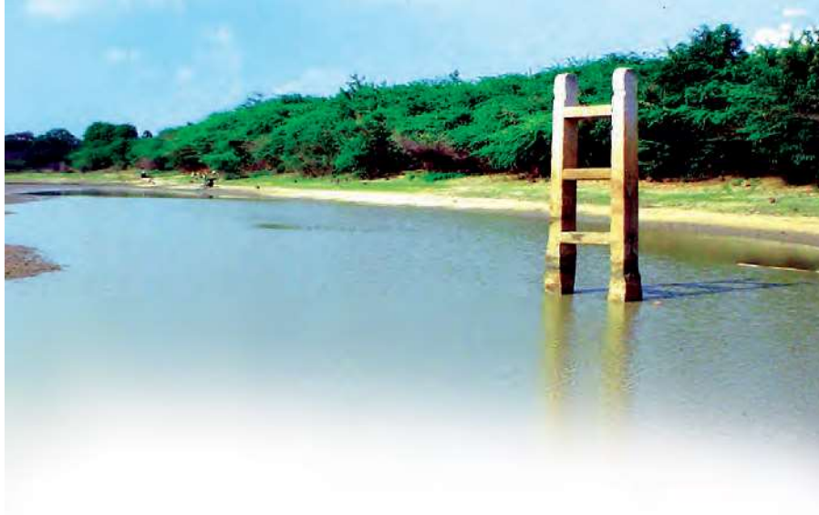
Fig. 5 A ninth-century sluice gate in Tamil Nadu. It regulated the outflow of water from a tank into the channels that irrigated the fields. A sluice gate is traditionally a wood or metal barrier which is commonly used to control water levels and flow rates in rivers and canals.
