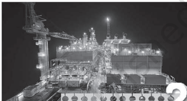
ONGC commencing its first oil production from Kakinada coast on January 7.
