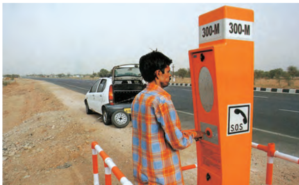
Fig. 7.10 : Emergency call box on NH-48
