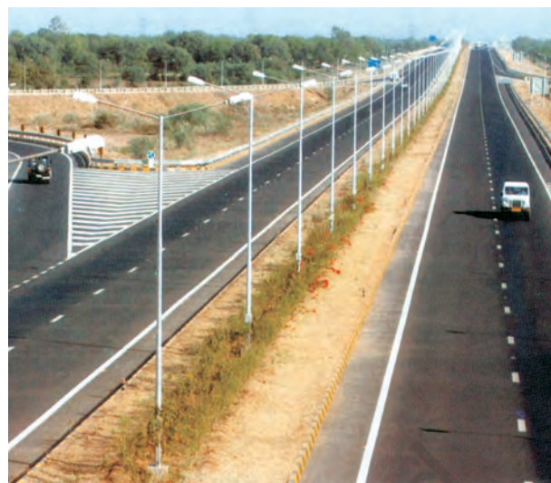
Fig. 7.2: Ahmedabad- Vadodara Expressway
