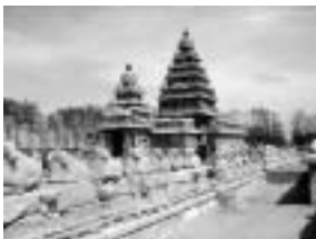
Shore Temple at Mamallapuram
