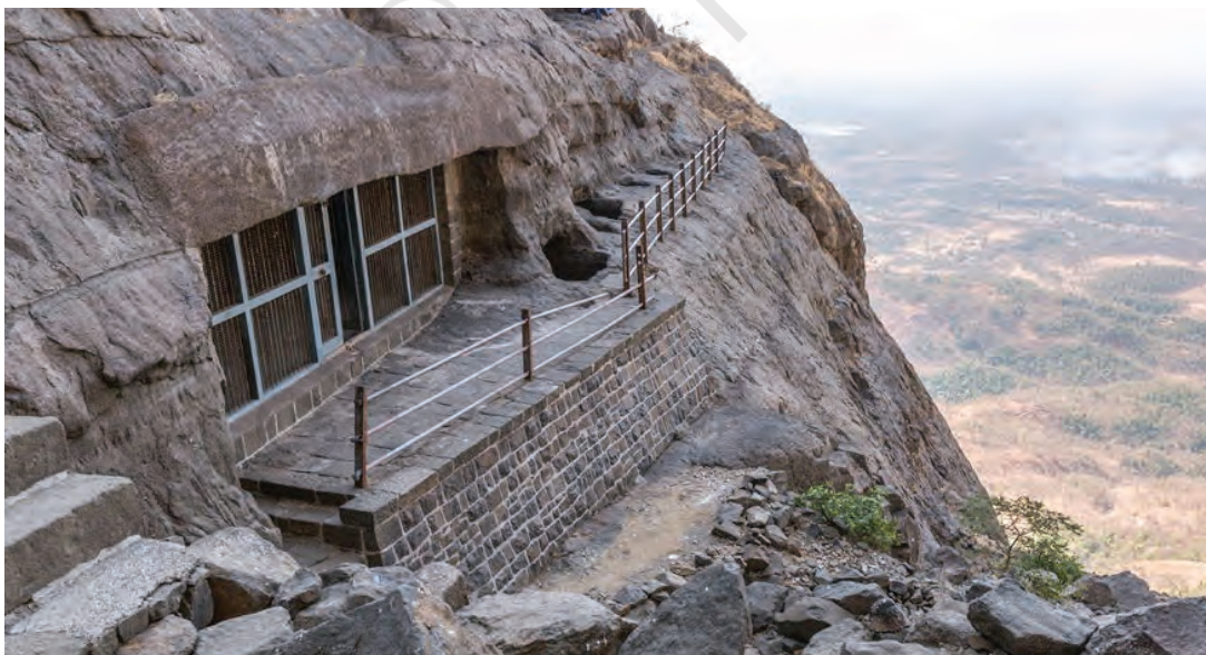
Fig. 6.9. The Naneghat Caves near Pune, located close to a major trade route, were used for collection of tolls and taxes, and as resting places for traders.
