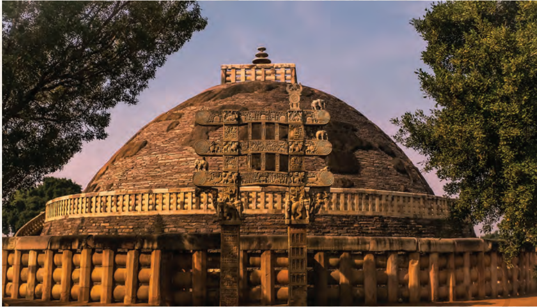
Fig. 5.26. As one of India's oldest stone structures, the Great Stūpa at Sanchi is among the finest examples of Indian architecture. Note that the original structure was made of bricks and was later enlarged using stone. Aśhoka is said to have constructed many such stūpas, chaityas, and vihāras for worship, study, and meditation.
